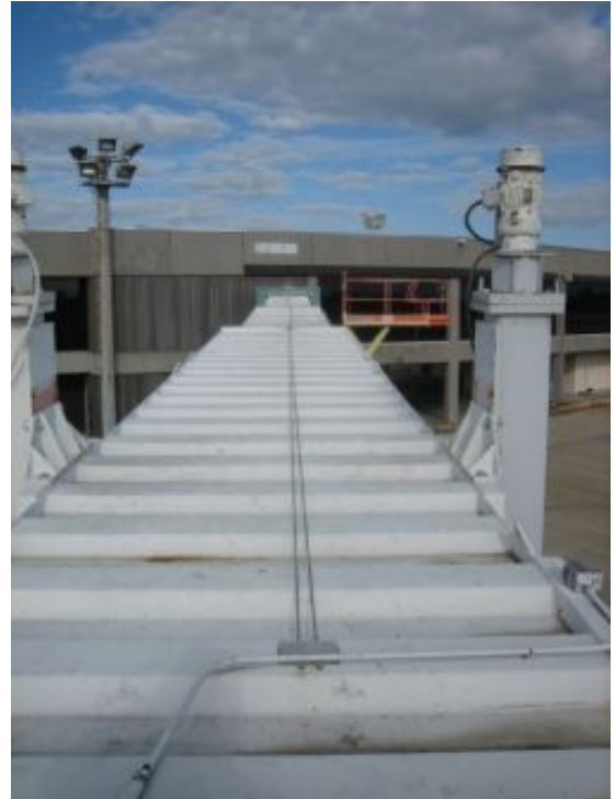
This device is a two cable lifeline with 4 bolt anchors on either end of each tunnel.
