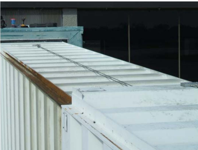
This device was a two cable lifeline with 4 bolt anchors on either end of each tunnel.
