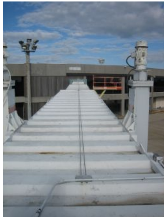
This device was a two cable lifeline with 4 bolt anchors on either end of each tunnel.
